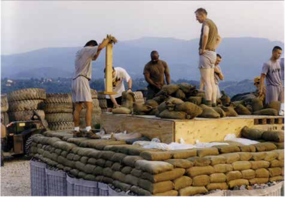
Figure 5-10. Force protection measures continued even without a direct threat. Here, MASH personnel build a sandbagged bunker, July 1996. Photograph courtesy of Lieutenant Colonel Steven Gouge.
