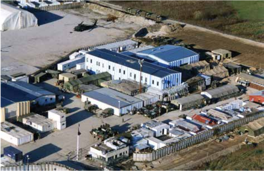
Figure 5-13. The Blue Factory, June 1996, with the Norwegian hospital occupying the buildings at the top left. The site would become somewhat more crowded when the 212th replaced the Norwegian unit.
